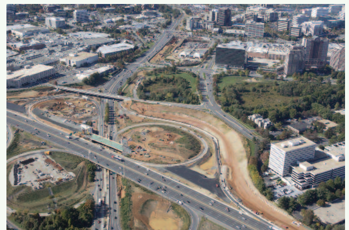
HOT Lanes and Dulles Rail construction
